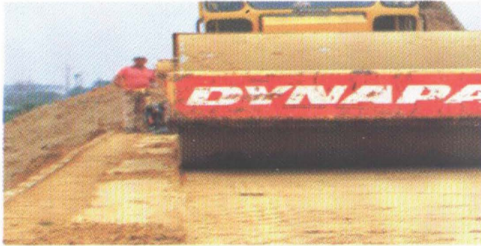
4) Compaction of the soil to 95% of the Standard Proctor.
