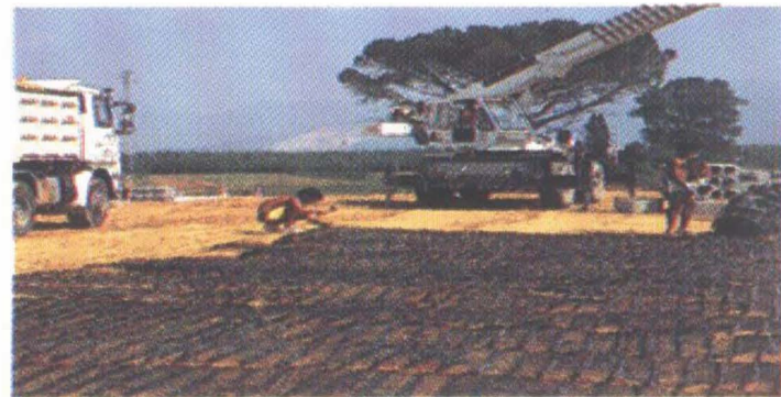
5) Laying of the Geogrids.
